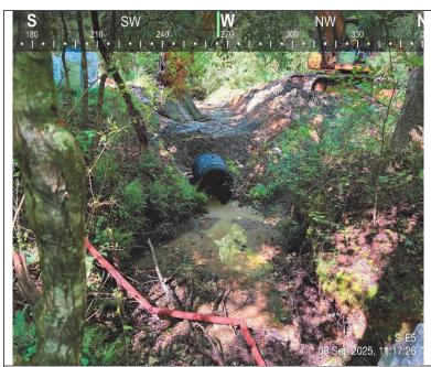
**Photo Description:** Culvert was replaced, countersunk, and backfilled properly. No impacts to biological conditions observed.
