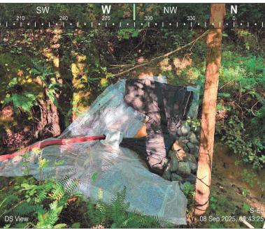
**Photo Description:** Discharge from pump around was filtered through a dewatering bag and filter stone.
