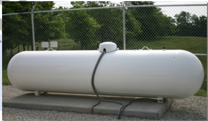
Propane tank dome protects the tank's fittings from damage and must always be in place.
