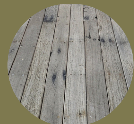
Bolt Holes Plugged ROUGH SAWN - NATURALLY GREYED OFF IN THE WEATHER
