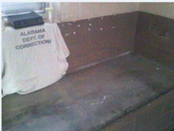
7c Concrete bed
