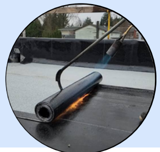
FLAT / TORCH-ON ROOFING
