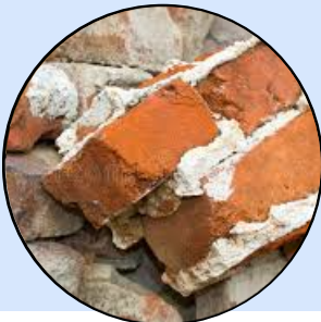
BRICK WITH MORTAR/GROUT
