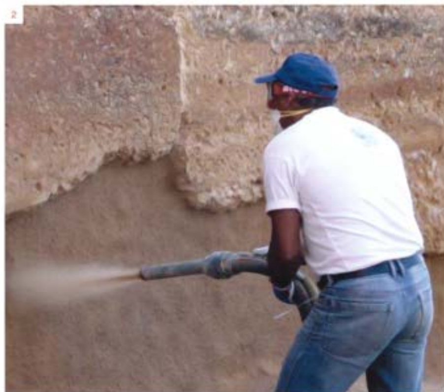
21 Sprayed earth: an innovative technique allowing for effective, durable and unexpensive rehabilitation of traditional raw earth constructions
