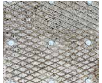
Attachment of wire mesh to concrete – distance to the wall to be lined: 5 mm / 0.19 inches
