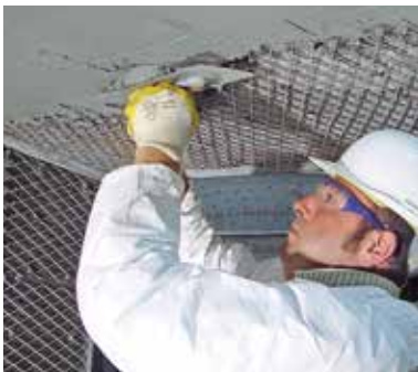
1. Overhead working is feasible without problem
