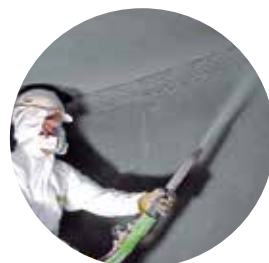
Spraying hose / spraying nozzle
