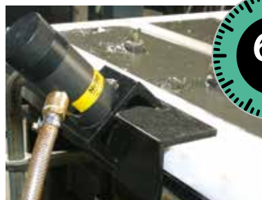
4. Use external vibrator for compacting
