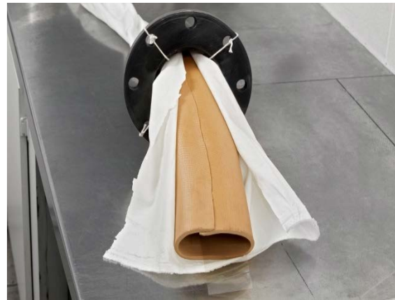
8, Pulling Tube through pipe with Cloth Liner
