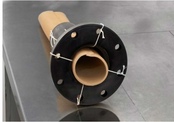
10, Expanding the tube against pipe wall
