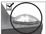
OVAL NECK OF BOLT SEATED PROPERLY
