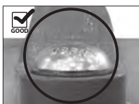
OVAL NECK OF BOLT SEATED PROPERLY
