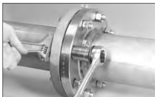
4-Bolt Tightening Pattern
