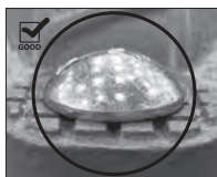
OVAL NECK OF BOLT SEATED PROPERLY
