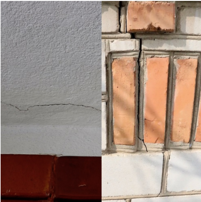
Cracks have appeared in recent years in residents’ homes close to the road, both on building exteriors and along the walls and ceilings of interior rooms.
