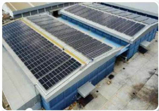
The roof of the original factory building.
