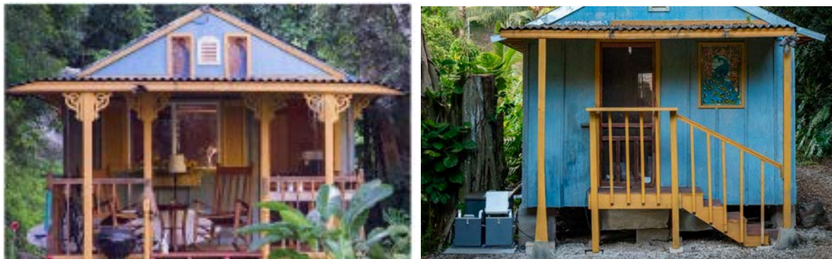
FIGURE 2.3: Site 2 household with 1 bedroom with 1 occupant (left) and mata installed to receive mixed wastewater (right).
