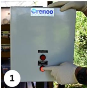
1 Press and hold Solids Change button until it beeps to start change.
