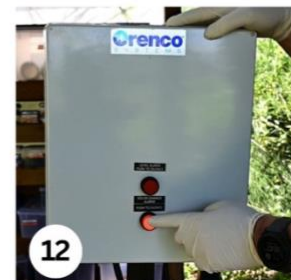
12 Press and hold Solids Change button until it beeps to end change.
