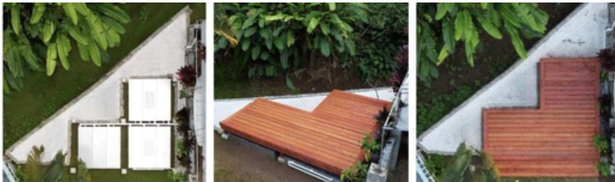
FIGURE 4.1 Sawa installation process
