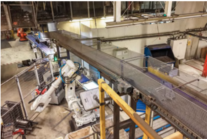
Shot Blasting System (1988) Schlick Roto-jet
