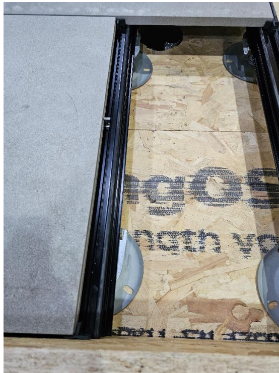
Plate 5 – Atria Porcelain Tiles Installed
