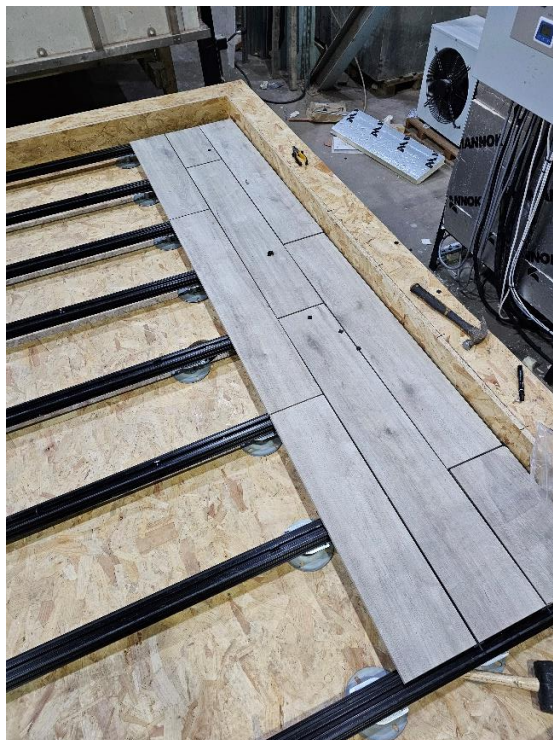
Plate 4 – Farrino Porcelain Decking Installed whilst Installing Pedestals
