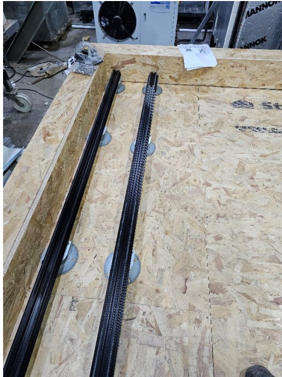
Plate 3 – Setting Joists and Pedestals Out
