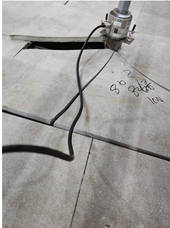
Plate 3 – Typical Failure for Atria Tile Point Load
