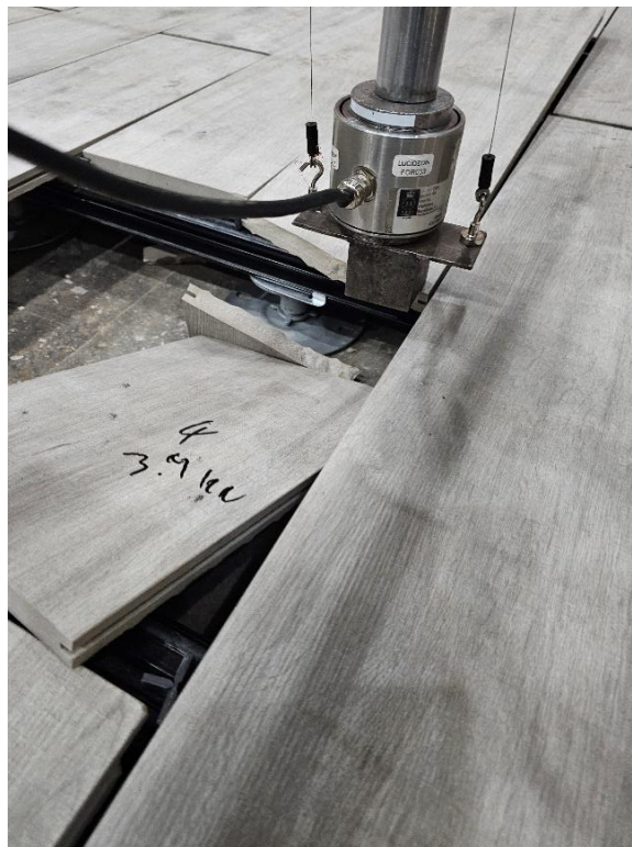
Plate 4 – Typical Failure for Farrino Tile Point Load
