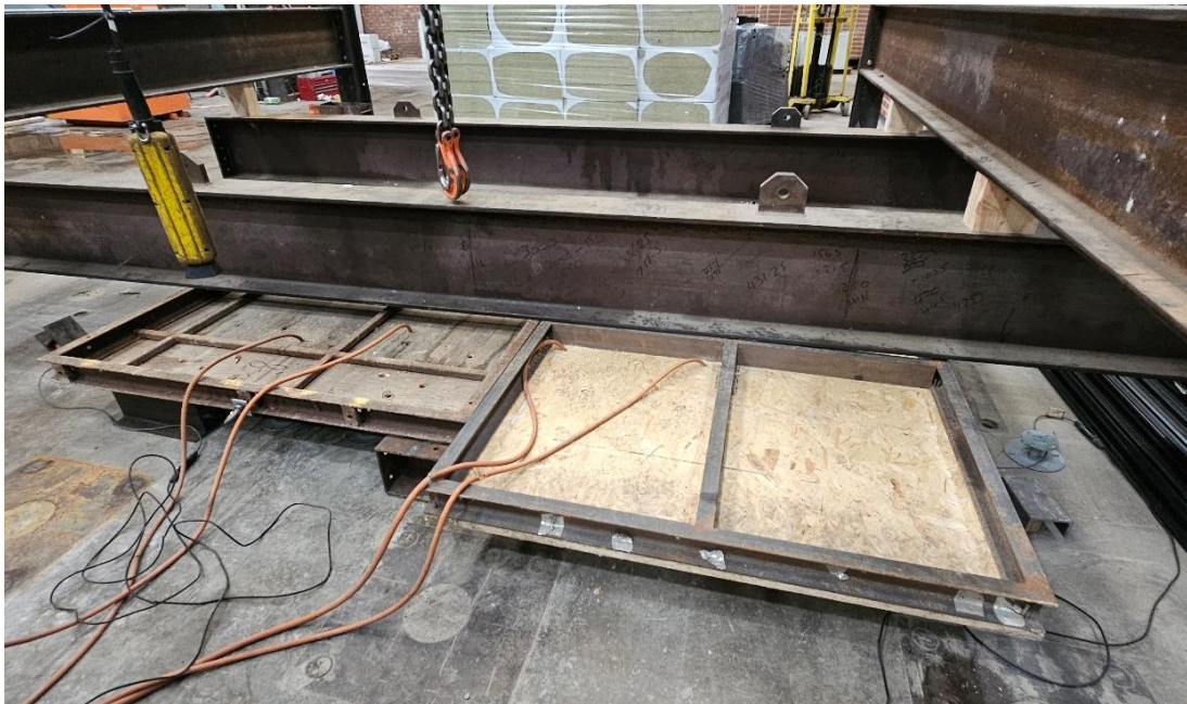
Plate 8 – Reaction Frames Installed
