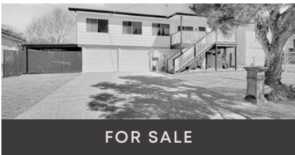
172 Matthew Street, Rosewood
