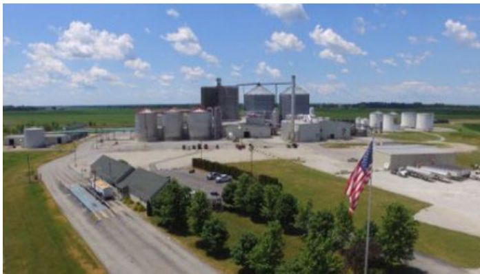
IBEC Facility (Rensselaer, IN)
