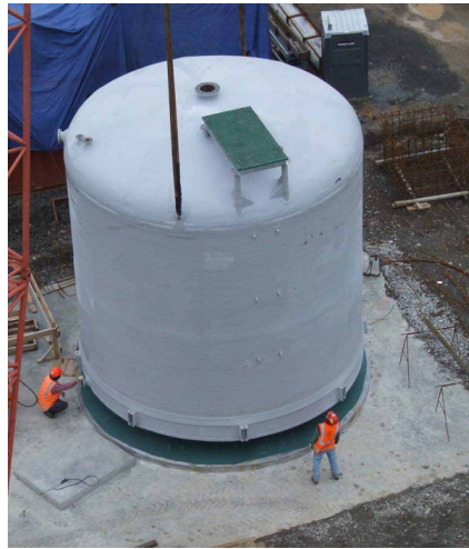
The areas where one needs to be careful and to use an appropriate catalyst level are usually found in the manufacture of flanges or where there is an overlap of two reasonably thick laminates.
