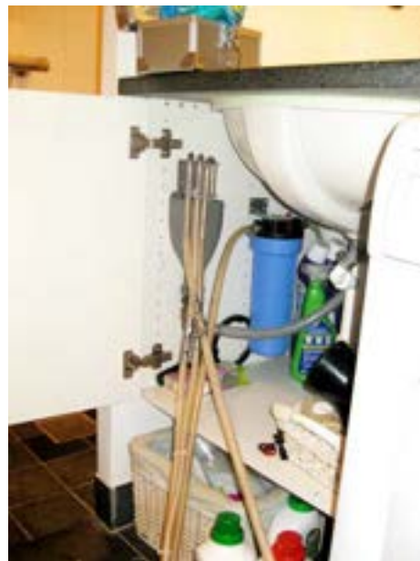
Figure 7. Water filter (photo courtesy of James Heaf).
