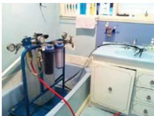
Figure 5. Examples of temporary water configurations. Home HD should not be excluded from those who have rental agreements that prevent permanent installation of fittings and equipment (photos courtesy of Anthony Perkins).
