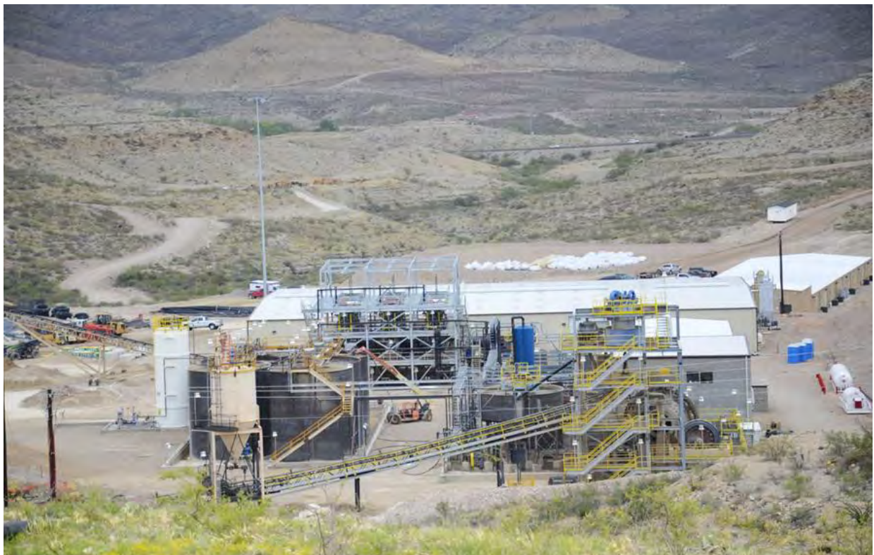
Figure 3: Shafter Processing Infrastructure.
