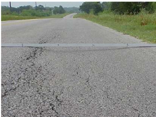
Figure 4.75 Rutting Example
