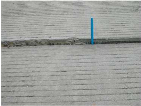
Figure 4.77: Faulting Example
