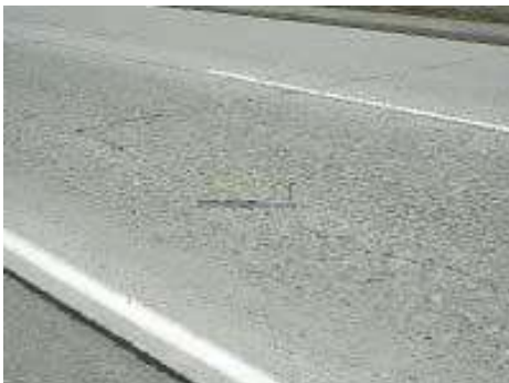
Figure 4.91: JCP Moderate Severity Longitudinal Cracking
