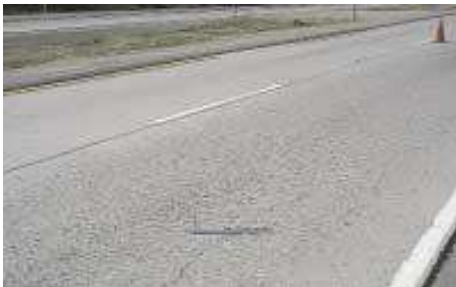
Figure 4.90: JCP Low Severity Longitudinal Cracking
