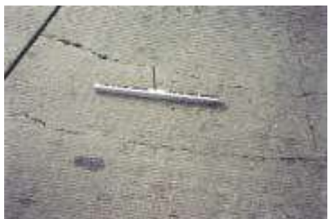
Figure 4.86: Low Severity CRCP Punchout Cracking
