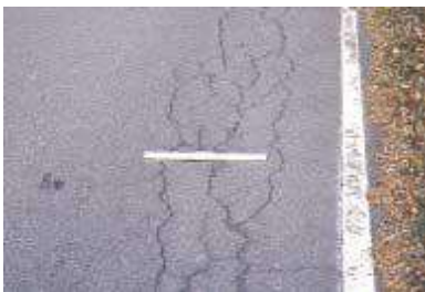
Figure 4.83: AC Moderate Severity Fatigue Type Cracking
