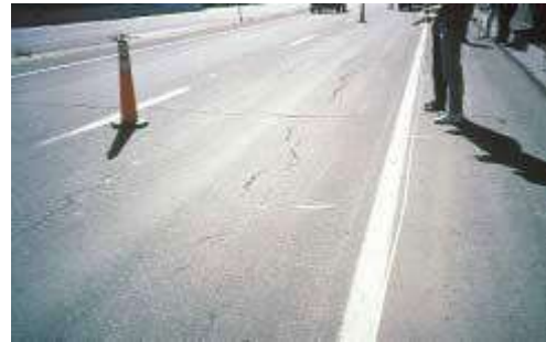
Figure 4.82: AC Low Severity Fatigue Type Cracking
