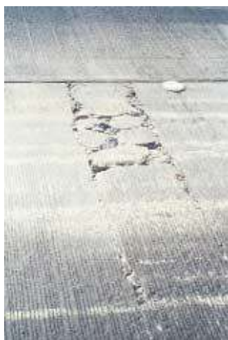
Figure 4.88: High Severity CRCP Punchout Cracking
