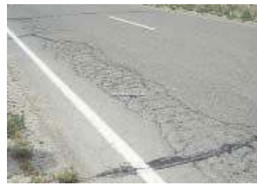
Figure 4.84: AC High Severity Fatigue Type Cracking
