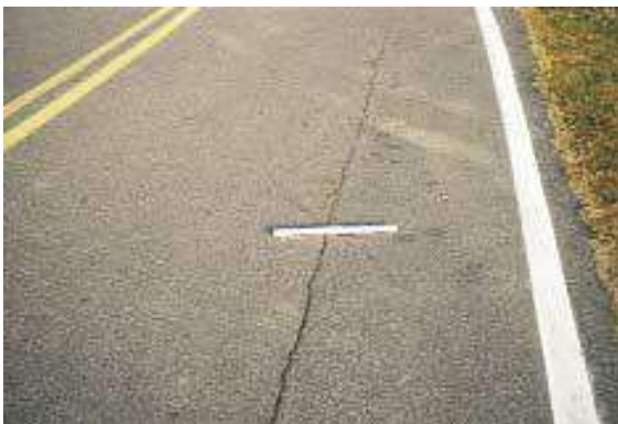
Figure 4.80: AC Moderate Severity Longitudinal Cracking (Wheel path)
