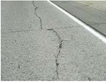
Figure 4.92: JCP High Severity Longitudinal Cracking
