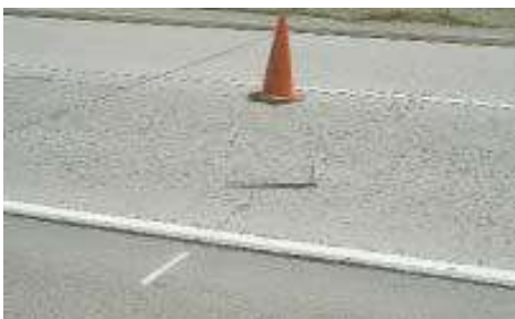
Figure 4.94: JCP Moderate Severity Transverse Cracking
