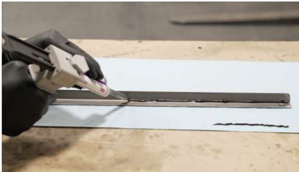
▲ Figure 60. Applying panel bond to support bracket
