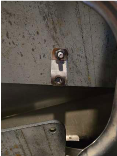
▲ Figure 29. Rear Middle Bracket installed
