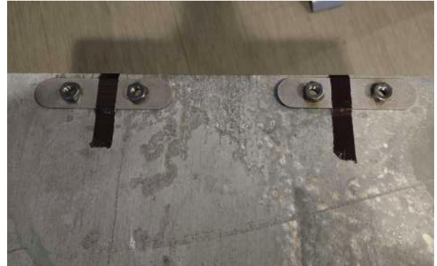
▲ Figure 27. Placing Pill Box Washers on back of the door using electrical tape
