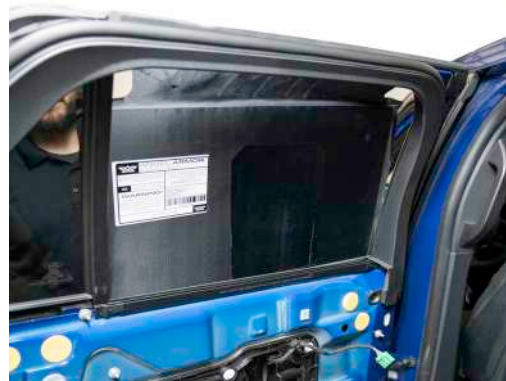
▲ Figure 19. Inserting the panel into the door.
