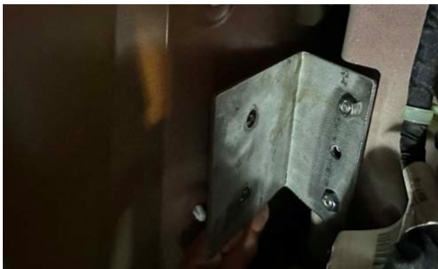
▲ Figure 36. Installing bolts with washers to lower bracket
