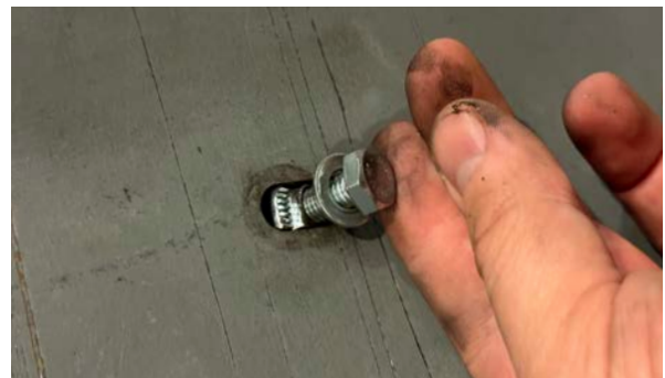
▲ Figure 37. Installing bolts through upper door armor
