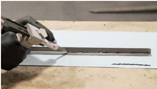
▲ Figure 64. Applying panel bond to support bracket.
