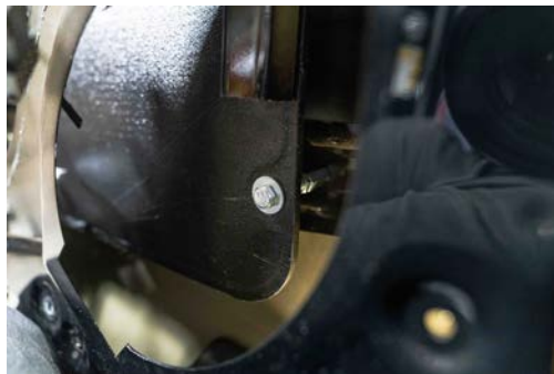
▲ Figure 69. Spacer Assembly Installed.
