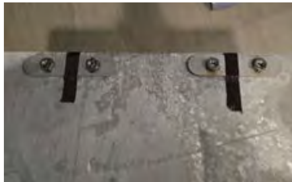
▲ Figure 27. Placing Pill Box Washers on back of the door using electrical tape
