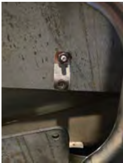
▲ Figure 29. Rear Middle Bracket installed
