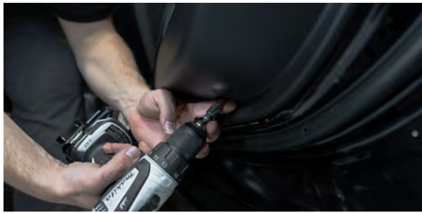
▲ Figure 26. Removing the lower panel bolts.
