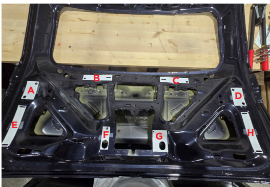
▲ Figure 29. Drill guides from Appendix A correctly aligned with their location on the vehicle hatch
