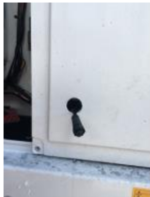
12-pin, straight device connector fed through the panel hole
