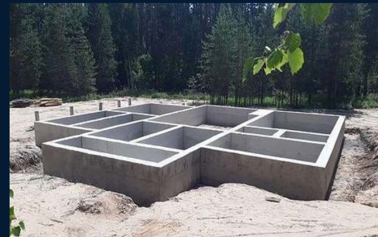
Pile binding with grillage/beam
