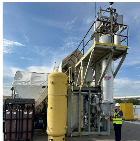
OxEon's Biogas-to-Oils (BTO) system, installed at Wasatch Resource Recovery's anaerobic digester, produced 128 gallons FT oil and wax.
