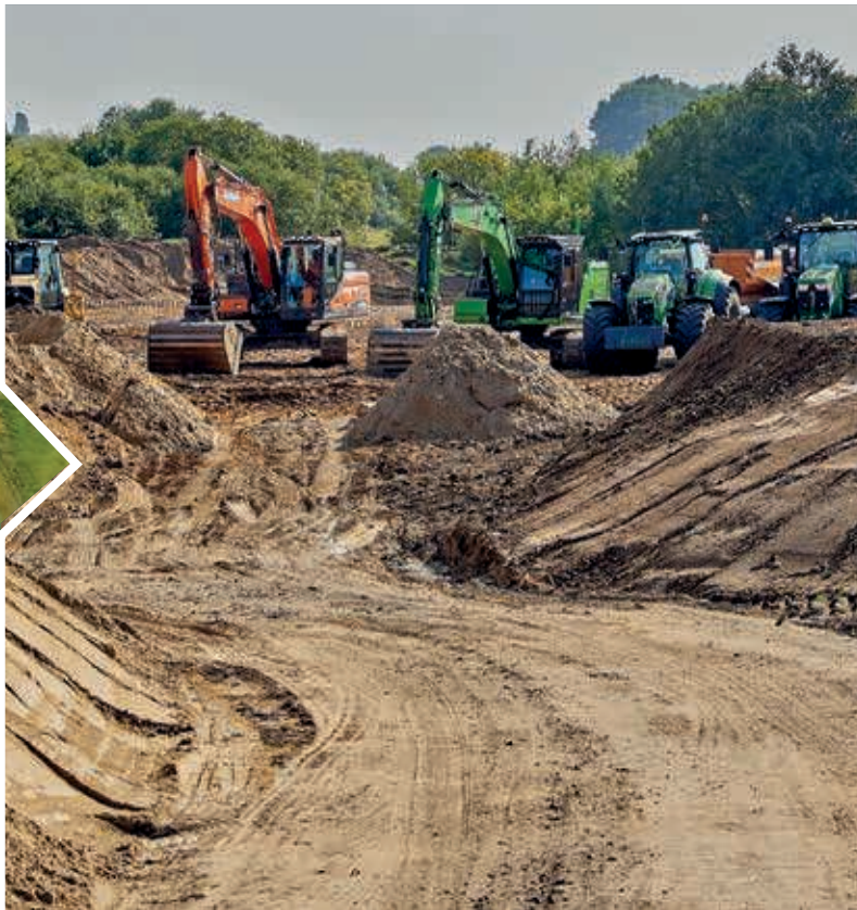
BAGGER IN ACTION ///
