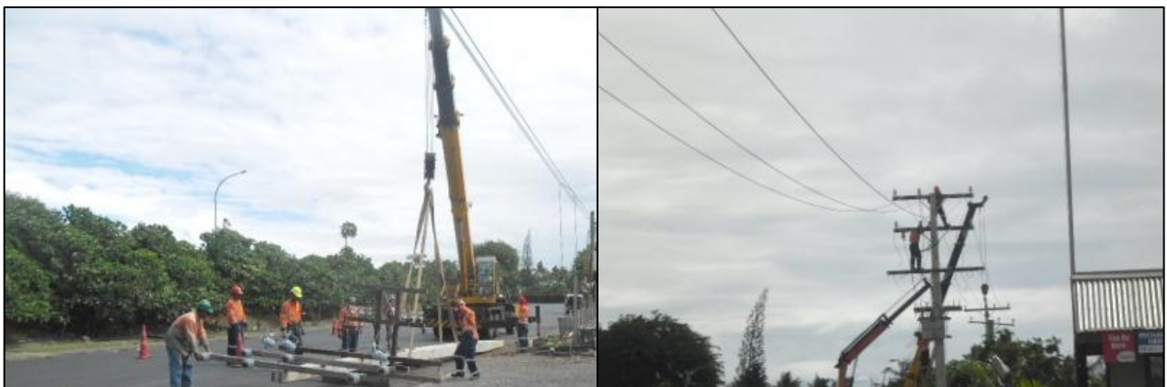
Above: EPC Linesmen Team at work replacing wooden with concrete poles within the Tuanaaimato area where the UN - SIDS Conference was held in September.
