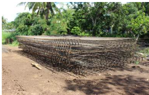
Rebar beams for the river wall foundation
