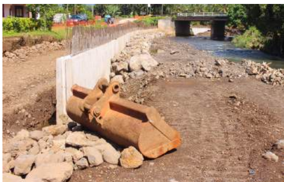
Construction of a revetment wall Vaisigano River
