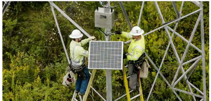
Image 2. Collection of still images from installation of LineVision sensor in AES Indiana
