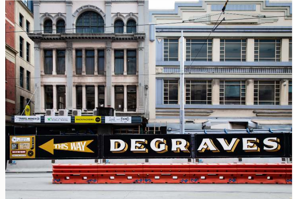
Top: Creative Signage by Weekdays Design Studio, Town Hall Station hoardings 2020
