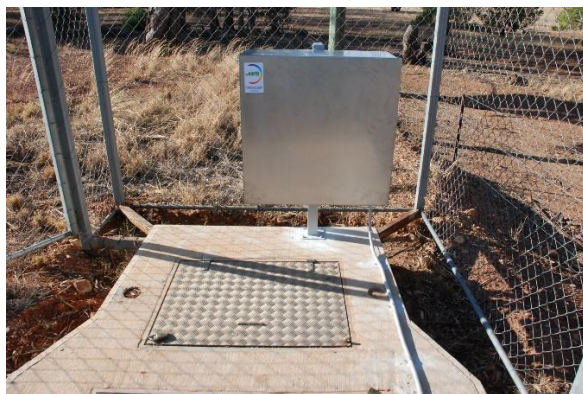
Left: Dosing pump plugged into 24hr power point timer. Below: S/Steel dosing cabinet
