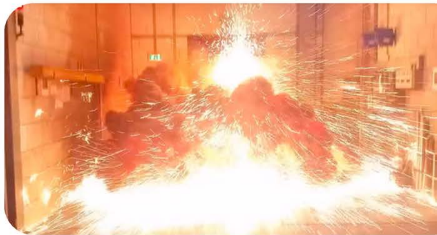
LOW VOLTAGE ARC FLASH EXPLOSION
