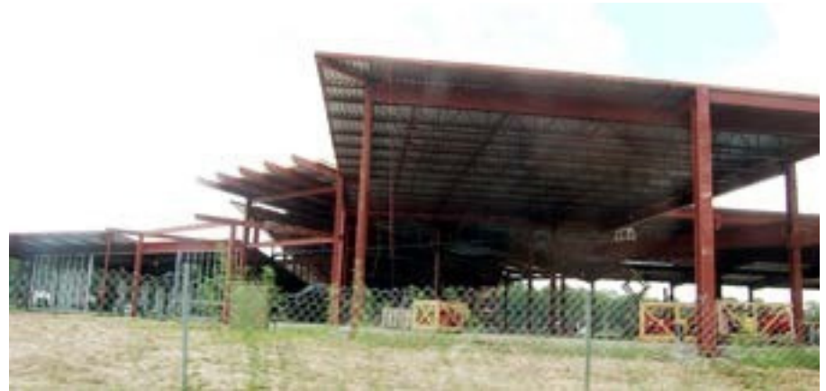
Ardendale site under construction in September, 2015
