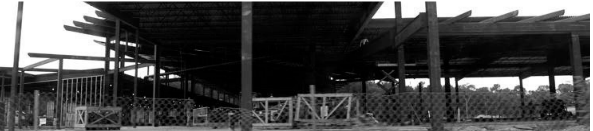
Ardendale site under construction in September, 2015
