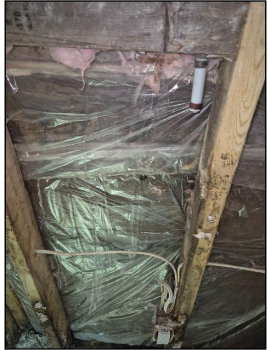
Drywall/insulation/vapour barrier cut back...
