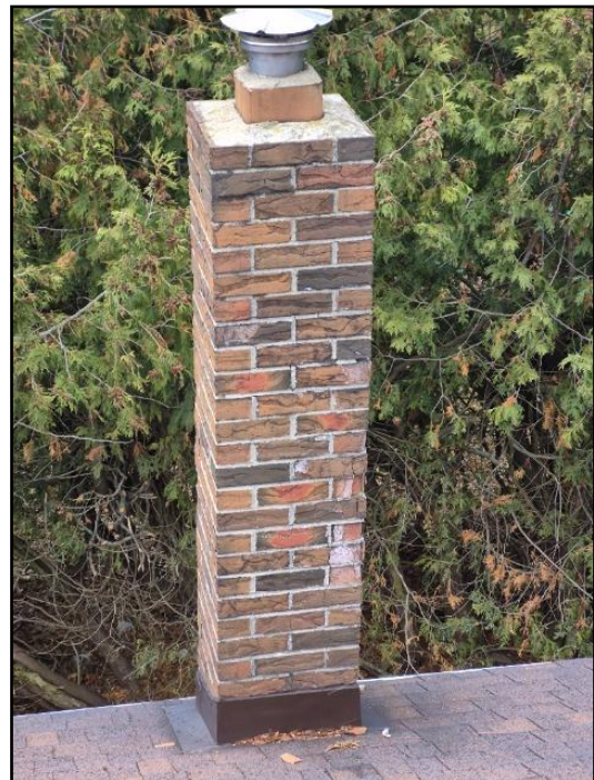
Masonry deterioration
