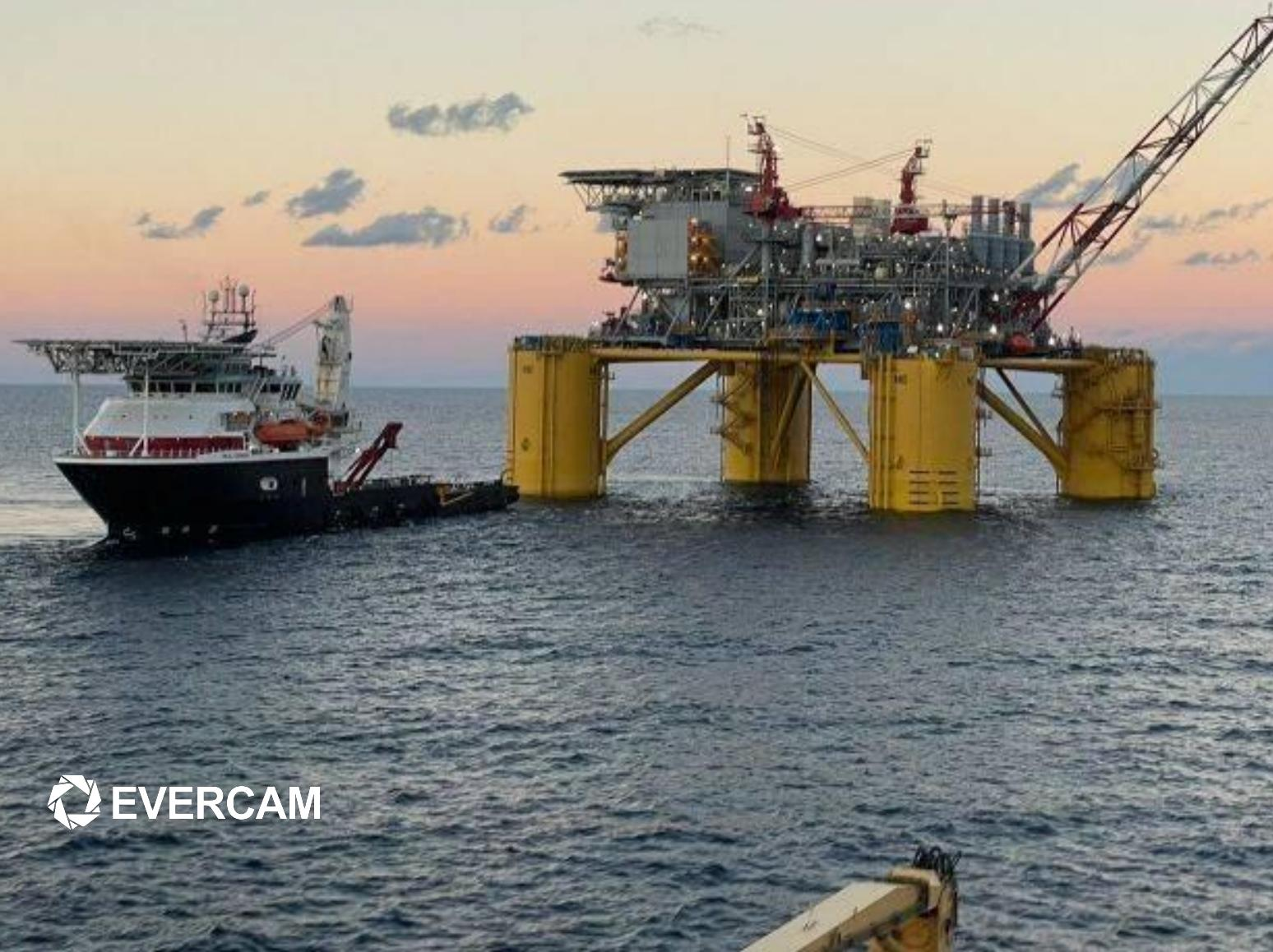
The Vito Waterflood Project in the Gulf of America is providing pressure support to the reservoir in order to increase oil recovery in the Vito field.
