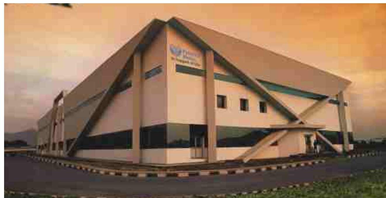
A view of manufacturing facility at Baddi
