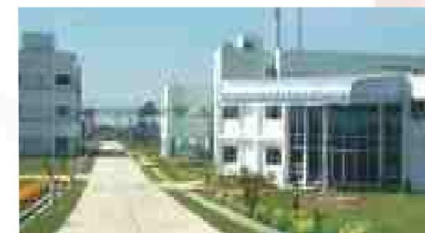
Recombinant Bulk Vaccine manufacturing facility at Lalru
