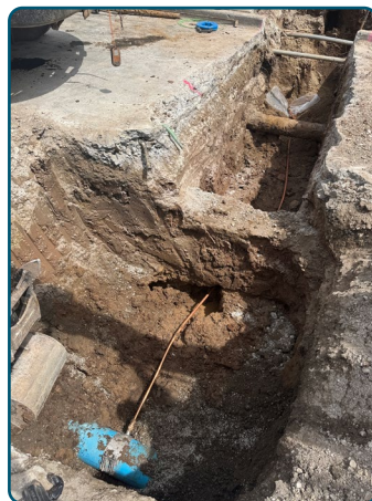
Water service line work on Oakland Avenue.
