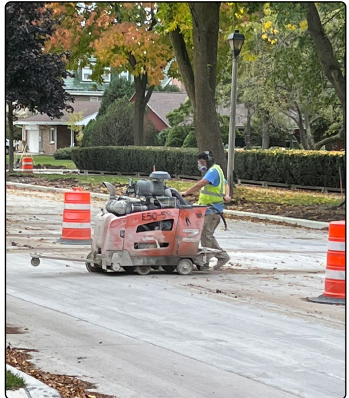
Pavement saw cutting
