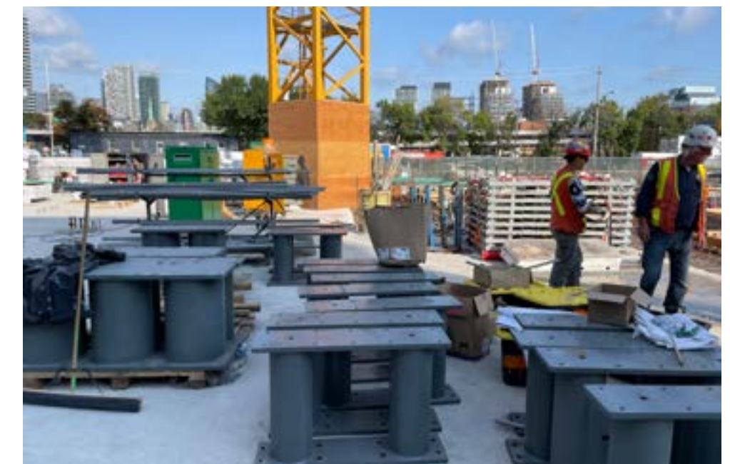
STEEL CONNECTIONS FOR THE MASS TIMBER COLUMNS DELIVERED TO THE SITE
