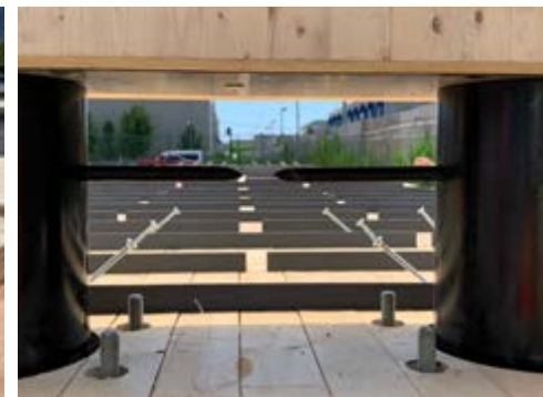
COLUMN TO SLAB CONNECTION
