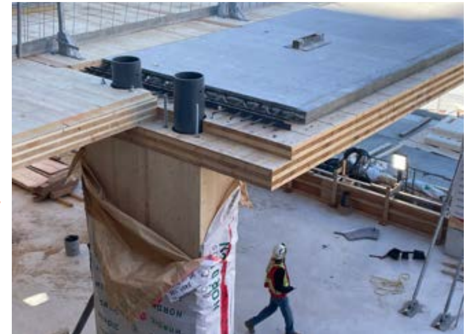
COLUMN TO SLAB CONNECTION
