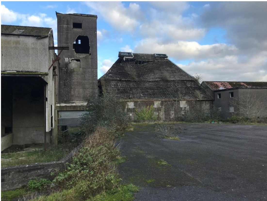
Southern Elevation Kiln Building & Malt House
