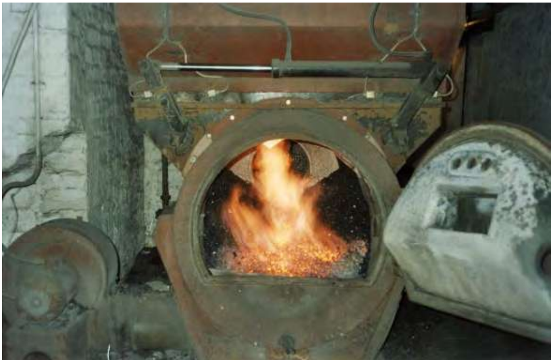
Fig. 18 Suxé anthracite furnace in operation in the Kiln house of the Village Maltings in 2001. Photo: Ursula O'Mahony.
