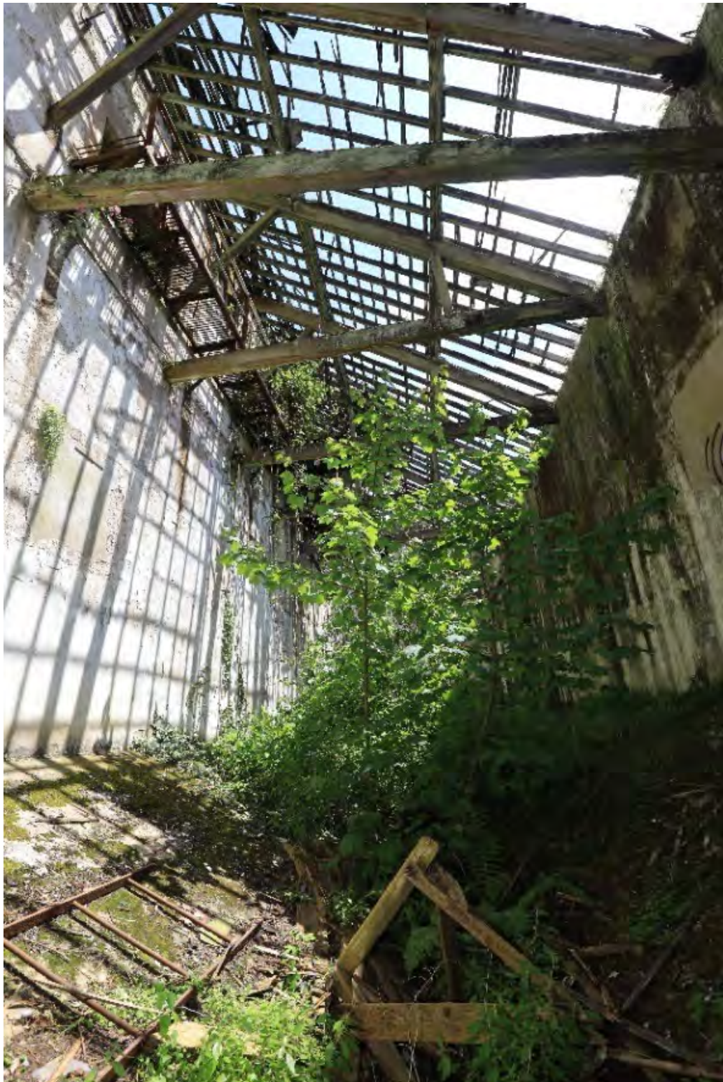
Fig. 74 Internal view of malt store, looking east, showing sloping floor and roof trusses.
