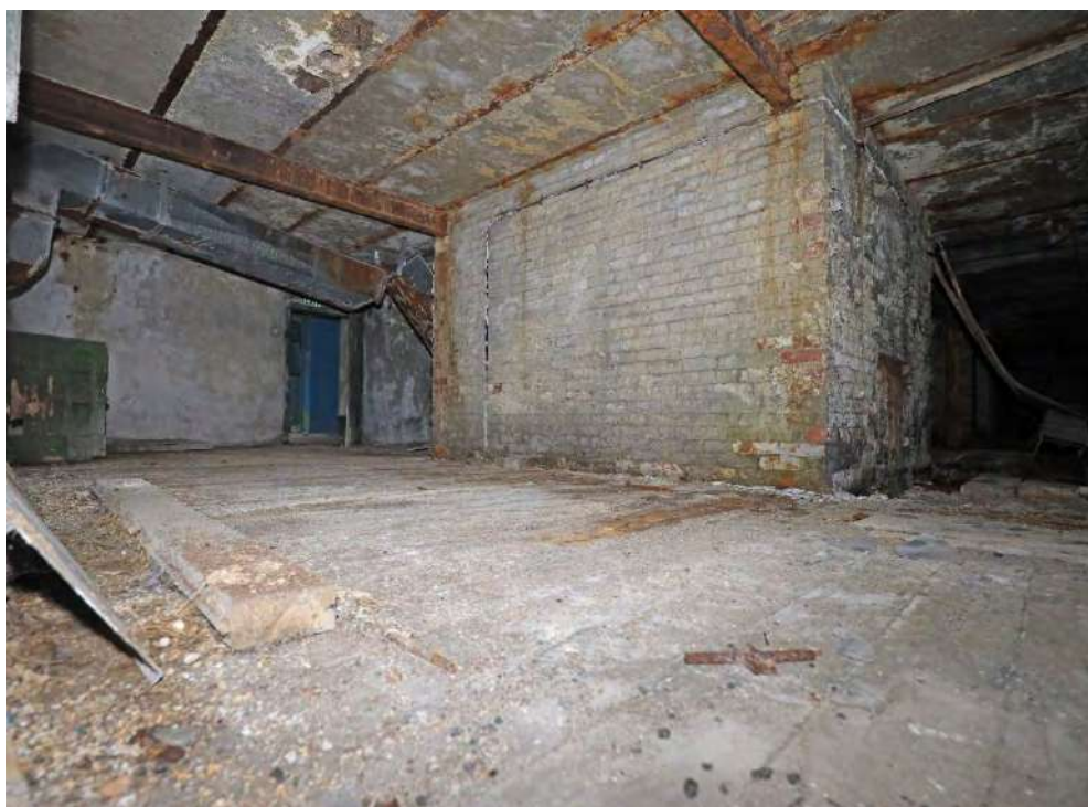
Fig. 71 Internal view of kiln house, showing supporting beams and brick flue (centre) leading from furnace to kiln floor.
