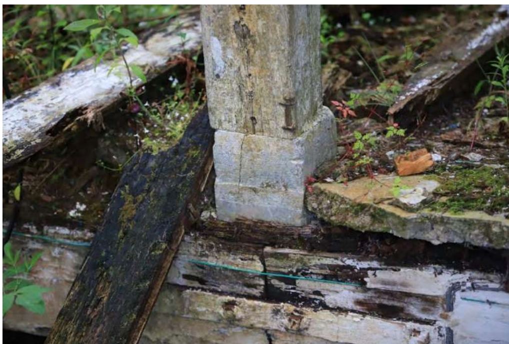
Fig. 60 Cut limestone padstone, supporting wooden stanchion at first-floor level in 1900s malthouse.
