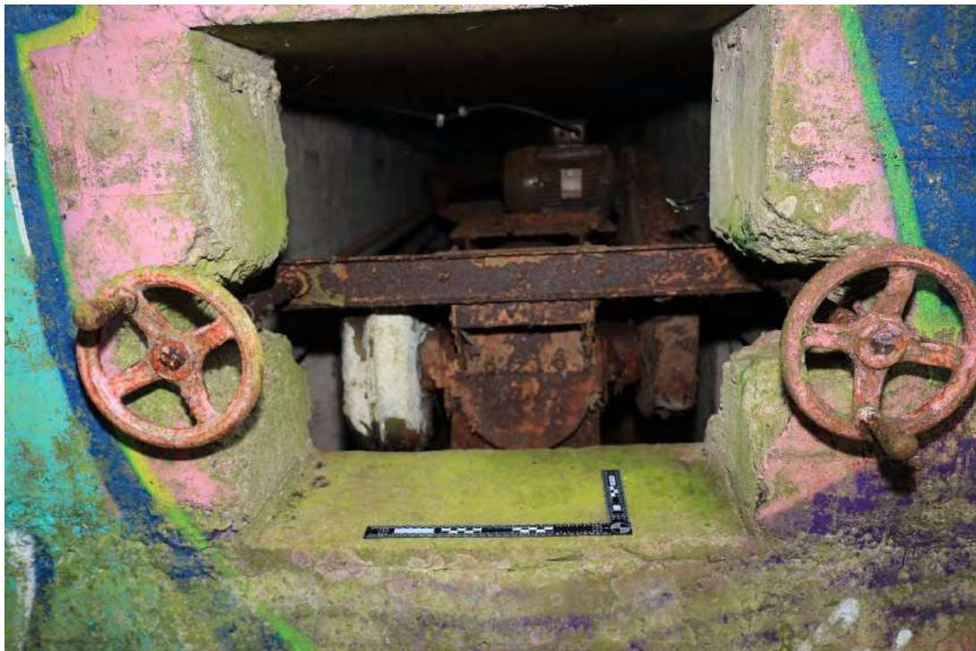
Fig. 86 Opening in south wall of grain silo for hopper regulator, shown here as crank-handled driving wheels.
