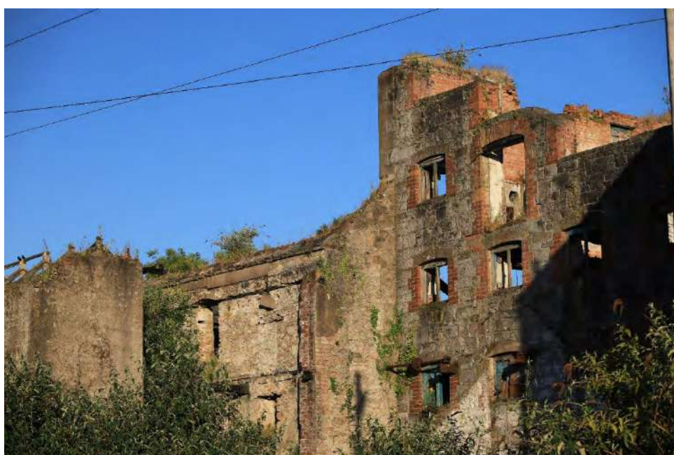
Fig. 52 Surviving portion of north-facing elevation of 1900s maltings, showing use of brick in upper storey.
