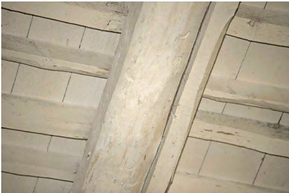
Fig. 34 Axe-dressed beams supporting loft floor, Smarts Store.
