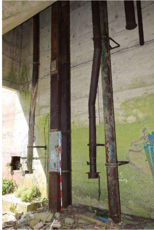
Fig. 85 Bucket elevator casing (left) and suction pipe (left), adjacent to east wall of silo.
