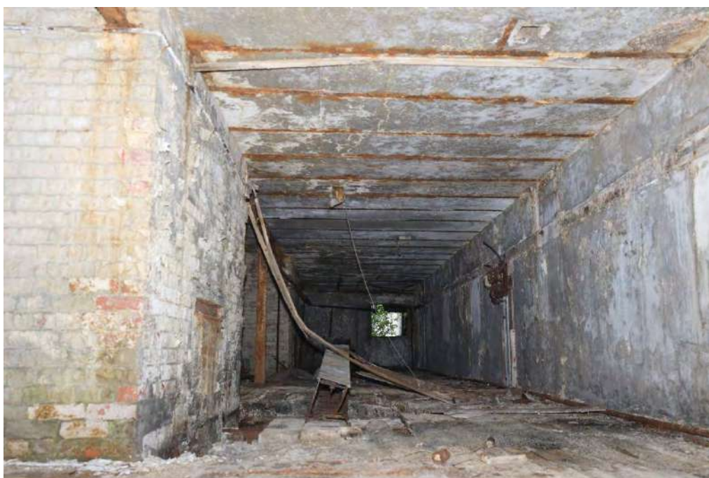
Fig. 72 Kiln house, looking eastwards, showing brick flues directing heat upwards from furnace on ground floor to kiln floor above.
