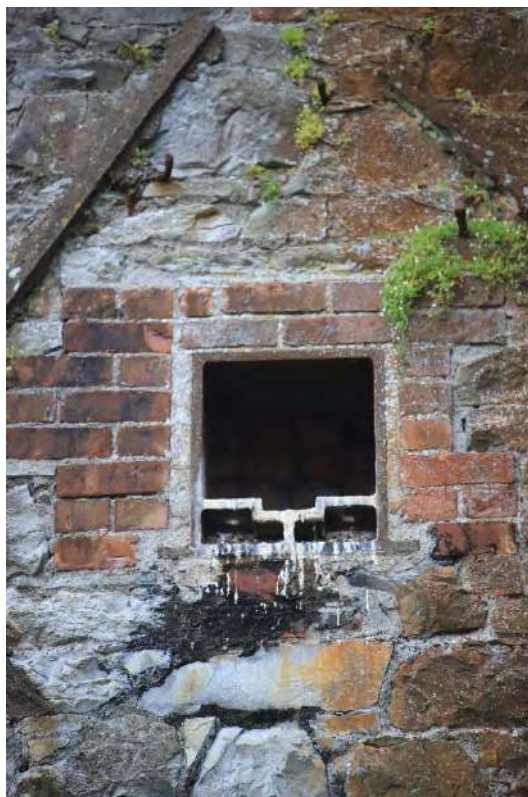
Fig. 69 Kiln house, west-facing elevation, 3 rd floor level, cast iron bracket for journal bearing.
