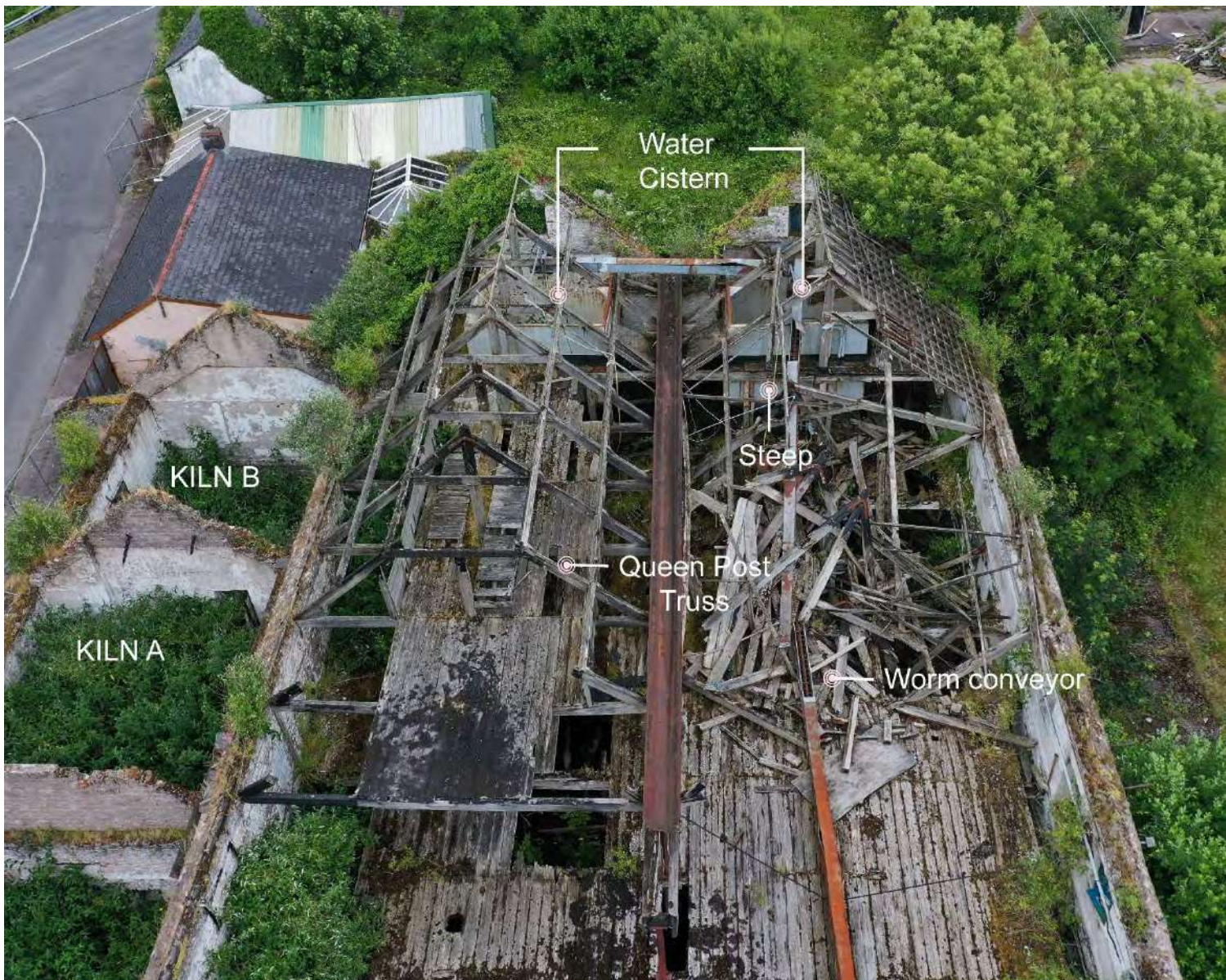
Fig. 48 Aerial view of ‘Old Maltings’, showing current condition (June 2024) and surviving machinery and plant.
