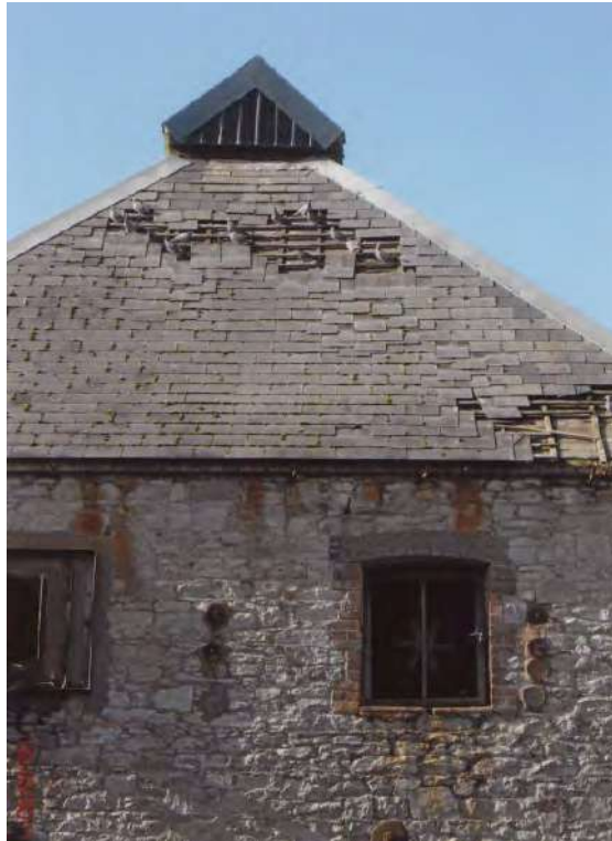
Fig. 68 Kiln house, east-facing elevation, showing tie plates.
