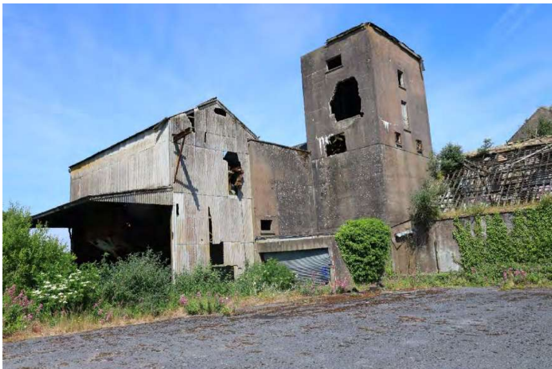
Fig. 84 1960s grain silo complex, south-facing elevation, showing elevator/hopper tower (right) and dryer house (left).
