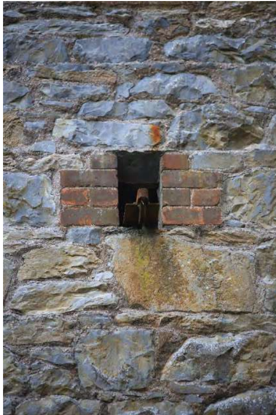
Fig. 70 Kiln house, west-facing elevation, 3 rd floor level, cast iron bracket for journal bearing.
