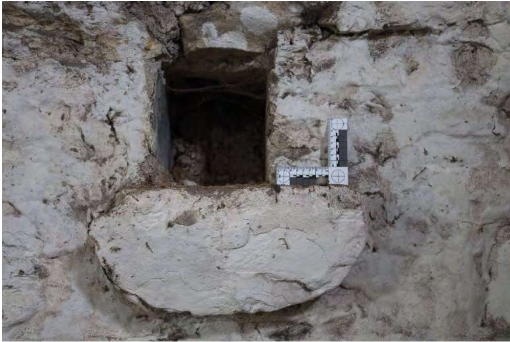
Fig. 33 Joist socket and stone corbel, north wall of Smart Store.
