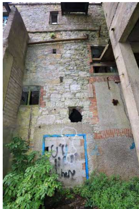
Fig. 67 Kiln house, access door for charging kiln with anthracite (right), from coal yard at west of kiln house.
