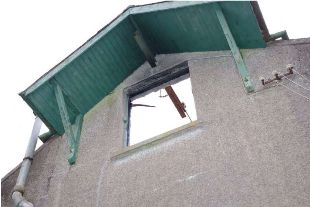
Fig. 79 Awning or lucamb , protecting sack hoist operations from the elements.
