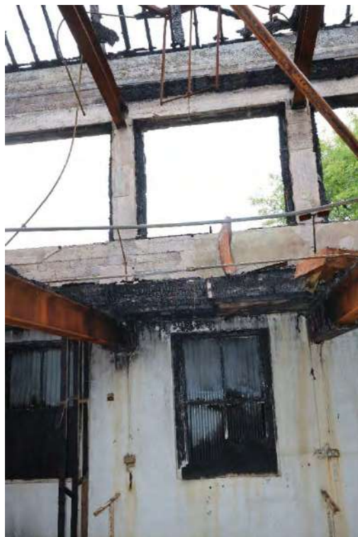
Fig. 80 Interior of laboratory extension, showing RSJs, supporting upper storey, and extent of fire damage.
