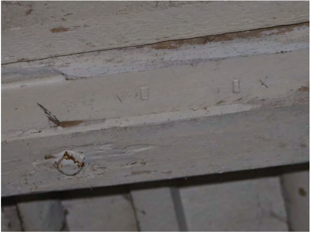
Fig. 35 Assembly marks ('V' and 'X') on cantilevered beam supporting loft floor in Smarts Store.
