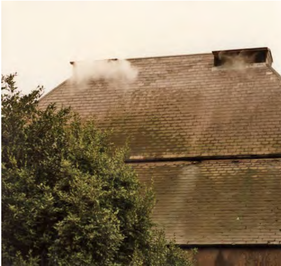
Fig. 17 Steam exiting louvred vents of Village Maltings kiln, 5 th December 1994. Photo: Kevin Dwyer.
