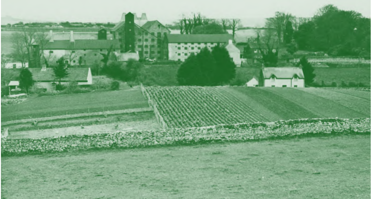
Fig. 39 The Village Maltings, c. 1940, looking east. The Northern Kiln house is on the extreme left. Kilns A and B are shown with shaft ventilators.
