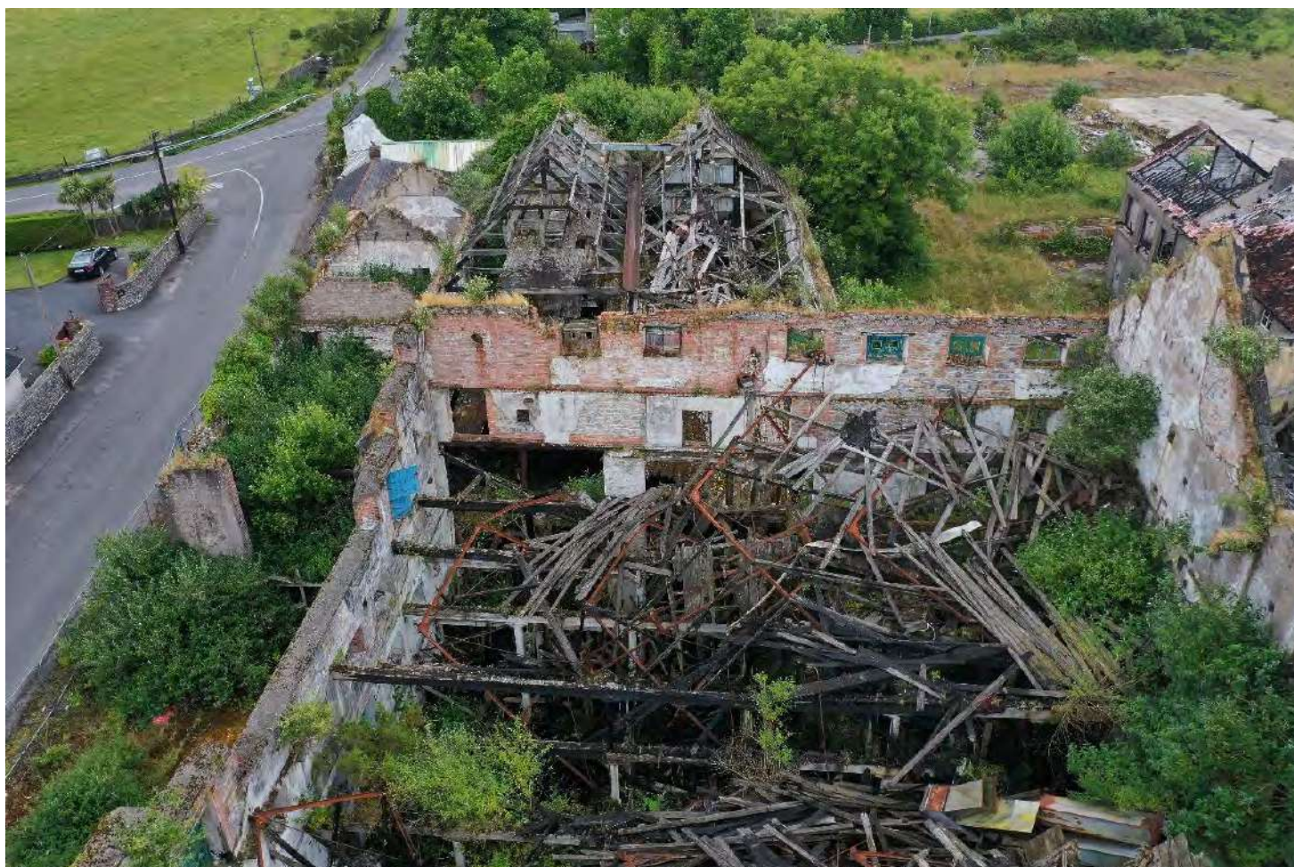
Fig. 51 Aerial view of 1900 maltings building. Note extensive use of machine brick in upper storey and on the apex of the gables.
